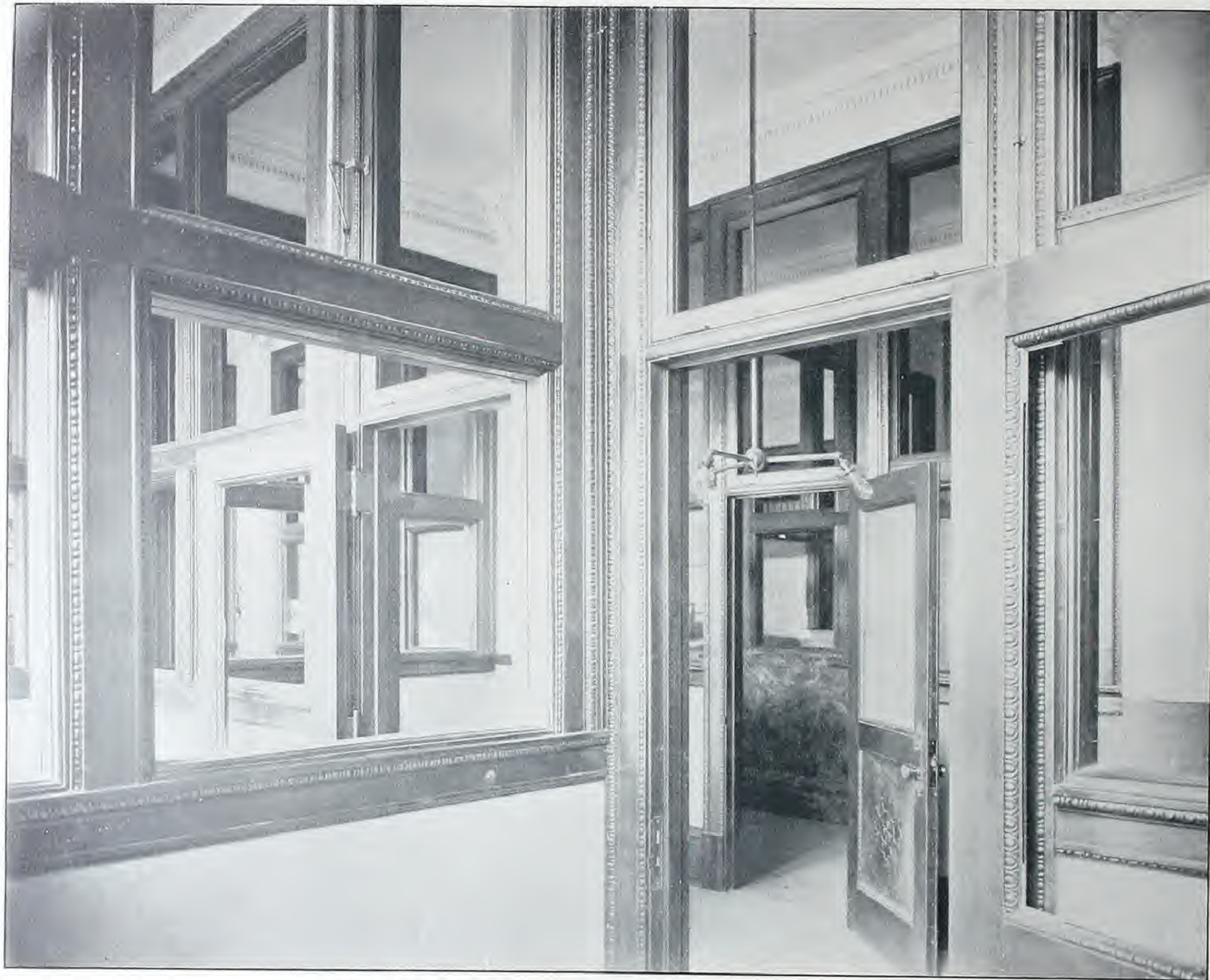
Fig. 147. —Interior View, Temple Building, Toronto.
